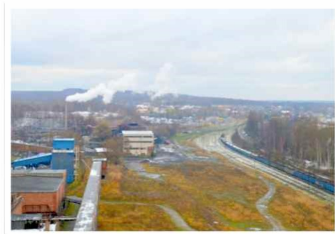
Figure 3 – Existing Site Facilities
