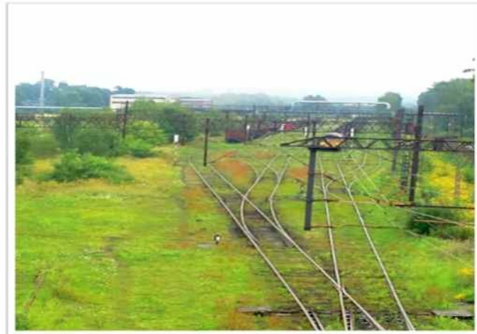
Figure 4 – Railway Siding at Debiensko
