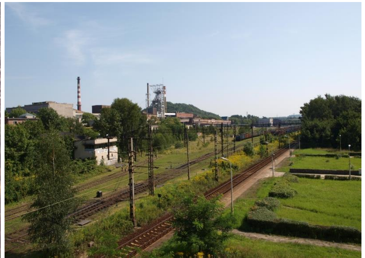
Figure 4 – Rail Yard at Debiensko
