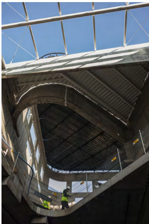
Galeria Młociny construction site, Warsaw
