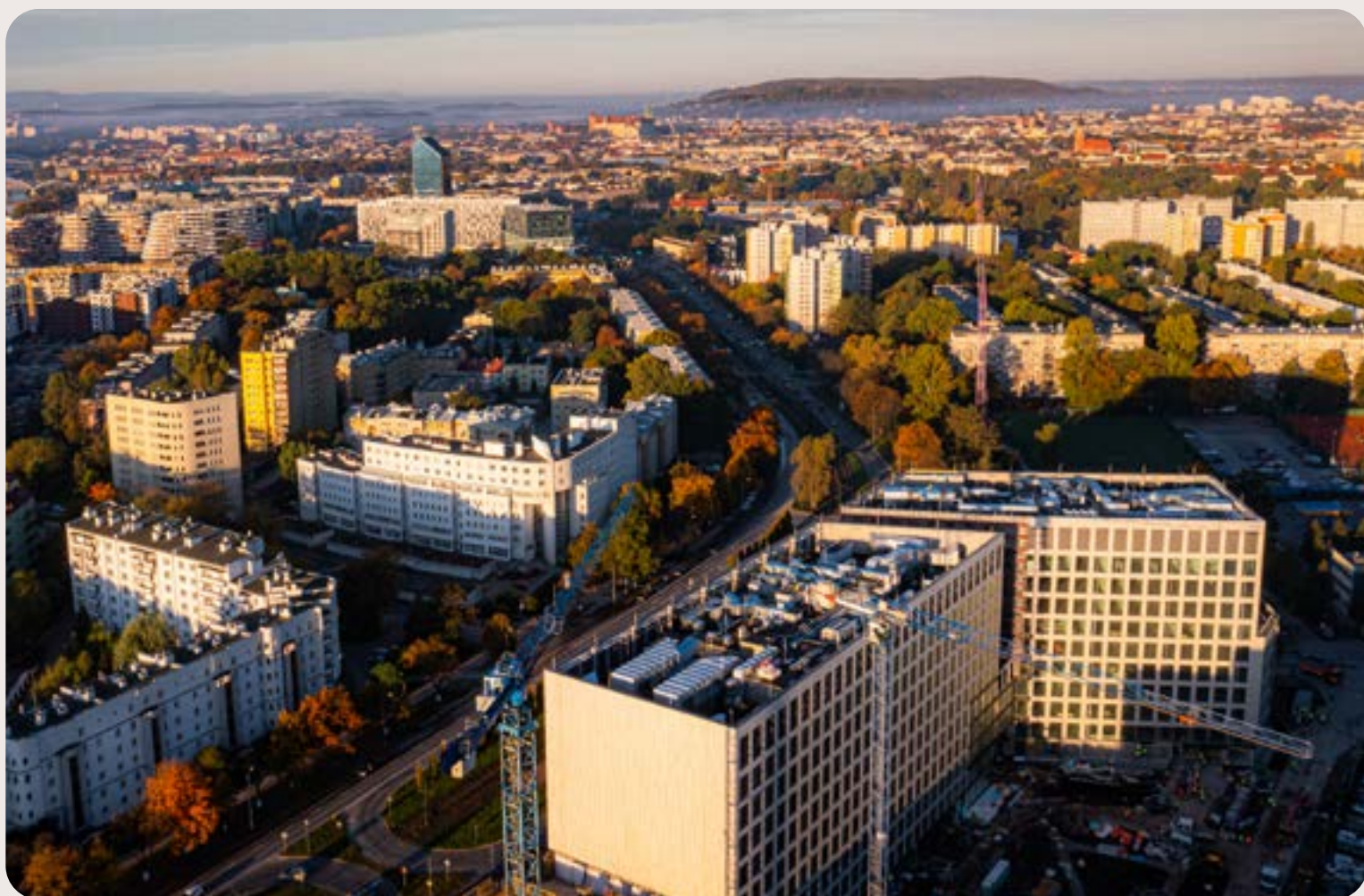
Photo: Brain Park office building in Kraków — under construction
