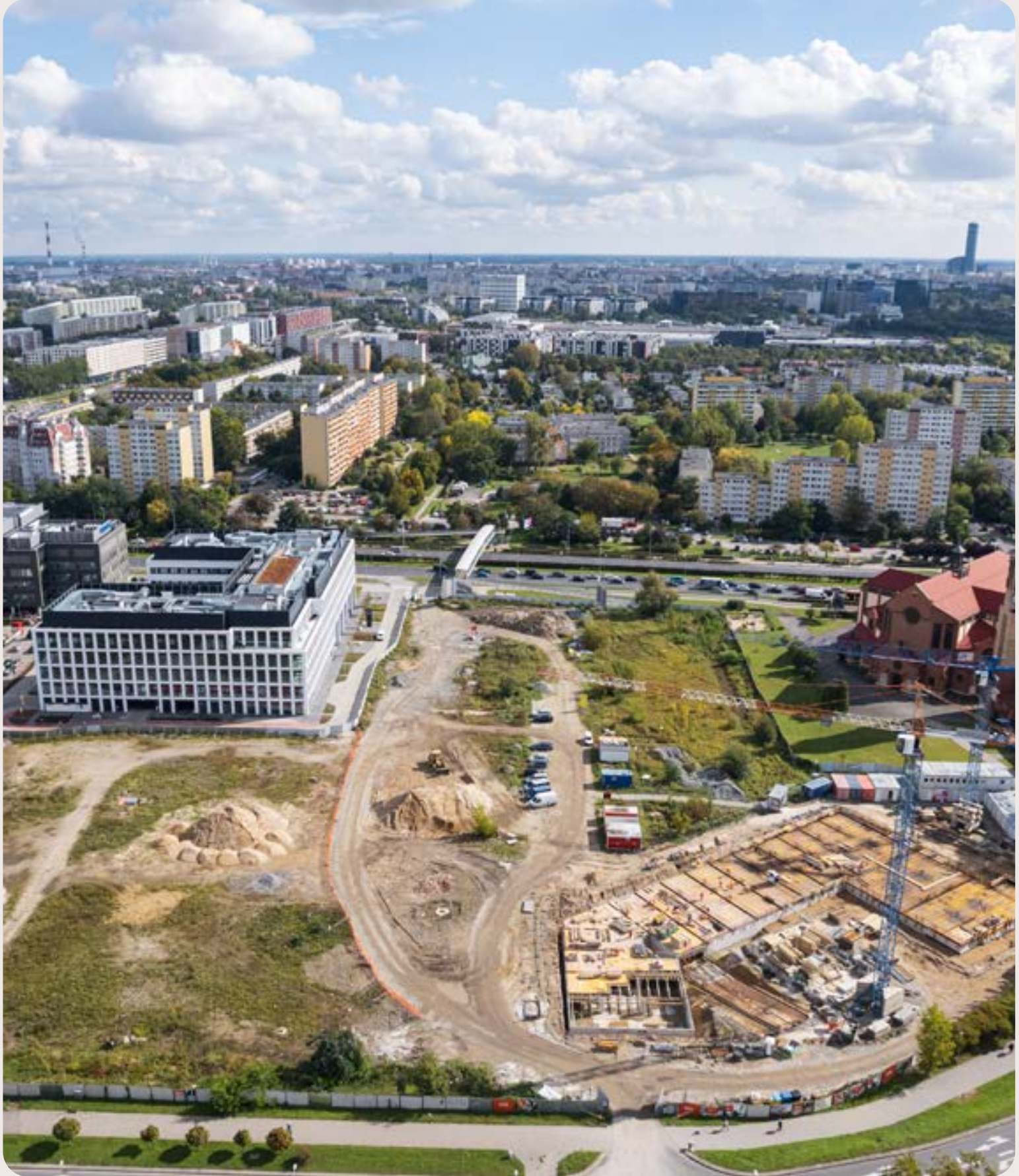
Photo: West 4 Business Hub building in Wrocław — under construction
